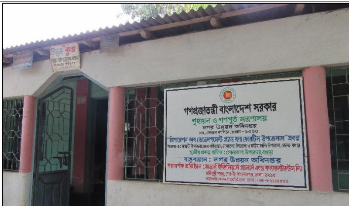
Pic 4. 2: Sonatola Site Office
